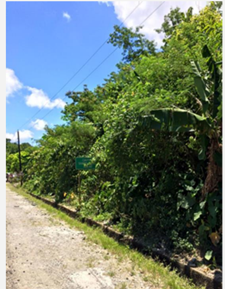
Obstructed Traffic Signs
