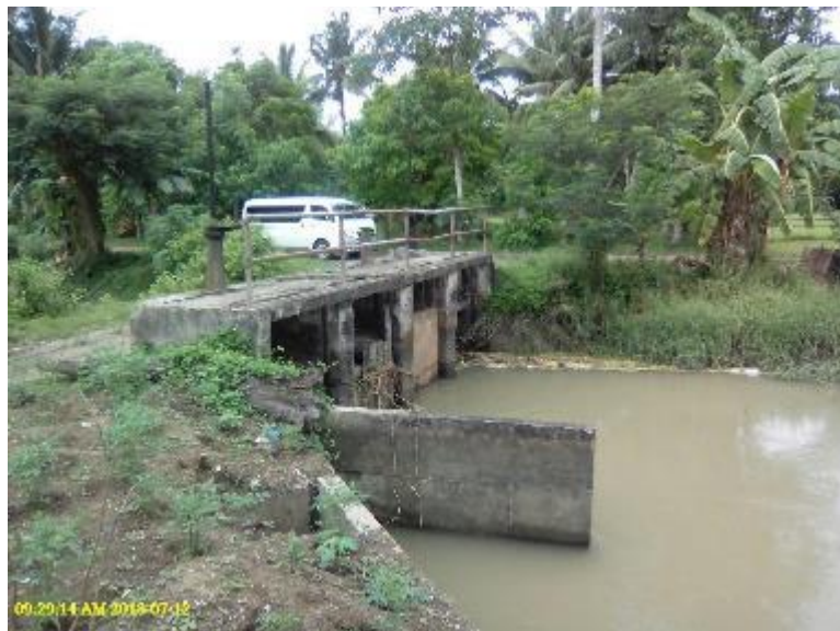
Photo 58. Check gate structure of Lateral B, Jalaar Proper RIS.
