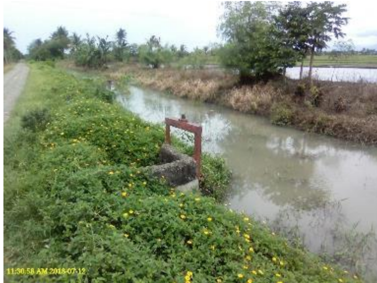
Photo 61. A direct turnout in the midstream of Main Canal of Jalaur Proper RIS.
