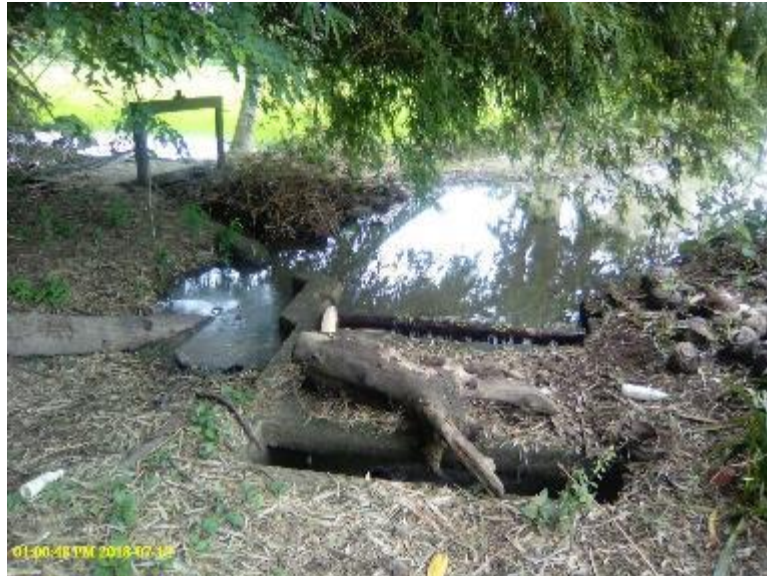
Photo 65. A re-use dam in Suague RIS. The intake gate is on the left side covered with debris.
