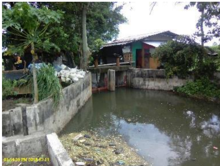
Photo 52. Checkgates at Lateral F, Jalaar Extension RIS. Take note of the floating debris on the left side.
