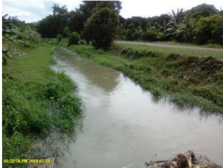
Photo 80. Main canal above designed water level in Padada RIS.
