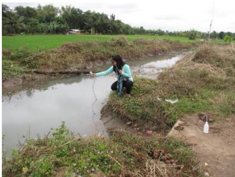
Photo 3. Damaged canal end section of Lateral D2-D2, Div. 4, MARIIS. Pile of sediments could be observed in both embankments of the canal
