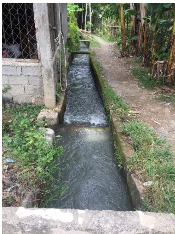
Figure 1B- 11. Main canal of Tagbawto CIS with width of 100 cm and height of 80 cm
