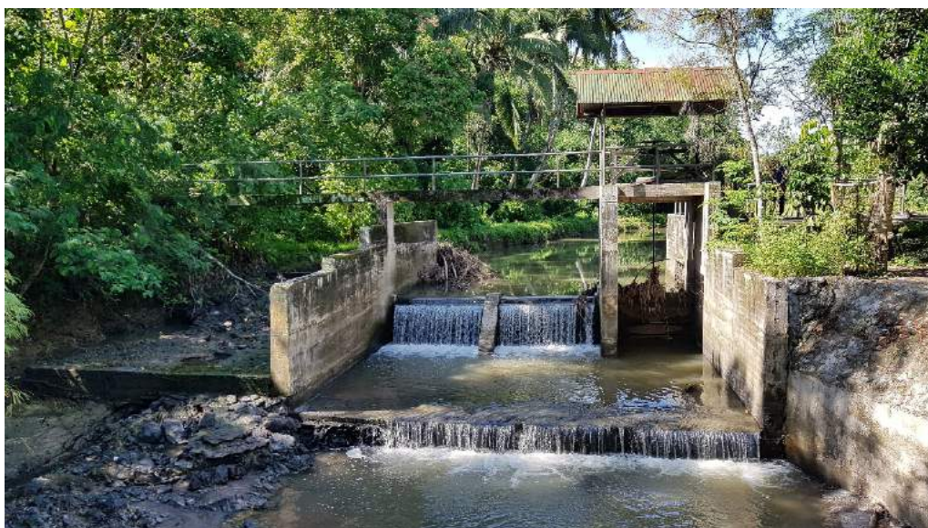
Figure 1C-25. The dam of Mani CIS with a sluice gate of 2 m width
