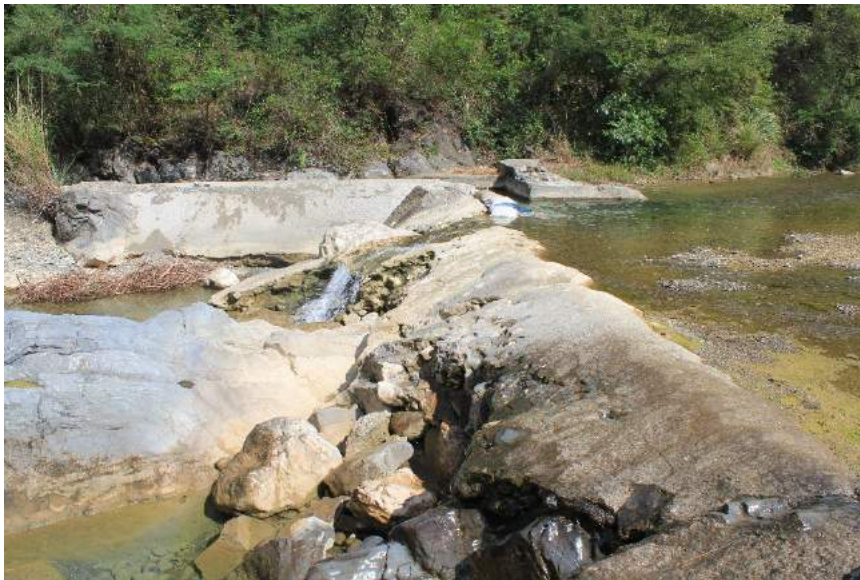
Figure 1A-36. The Parang-Bugnan CIS dam; the damage at the ogee spillway exposes the dam core made of rocks and boulders; the sediments are almost at the dam crest level
