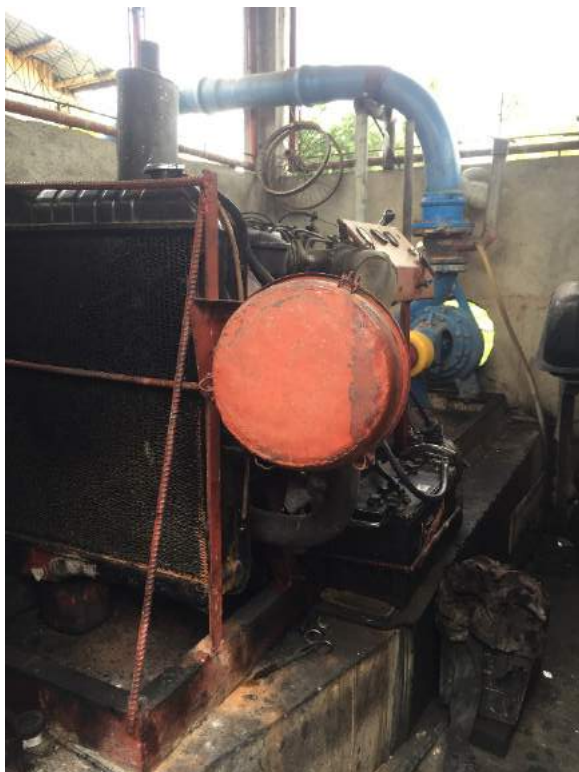
Figure 1B- 35. The centrifugal pump and the diesel engine of the Sigma Sur PCIS
