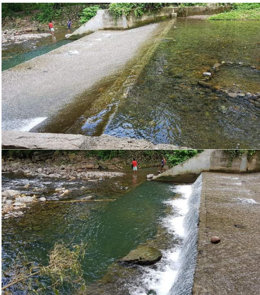
Figure 1C-1. Marapangi Dam of Unifarm CIS showing sedimentation and damaged downstream apron of the dam
