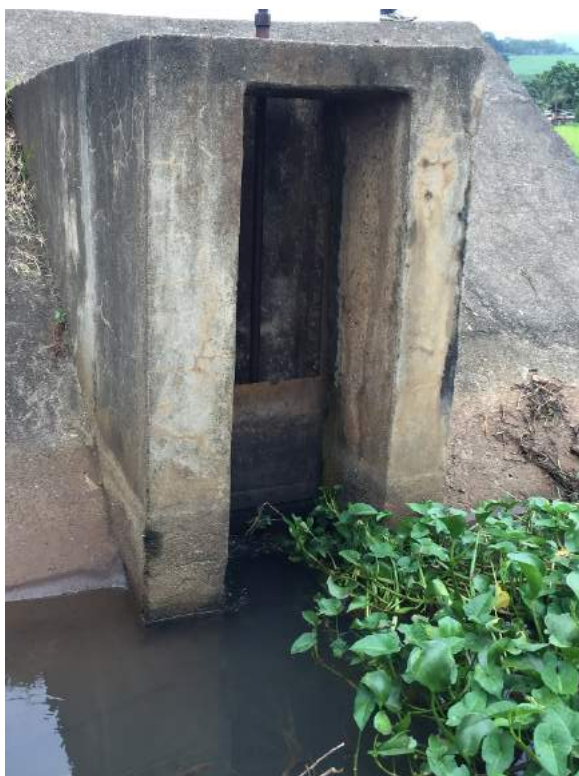
Figure 1C-38. Right main canal intake with 0.5 m width
