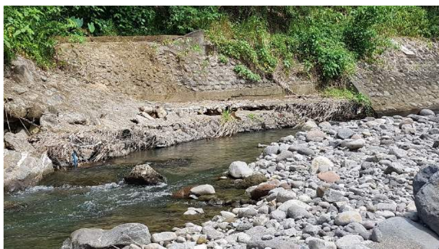
Figure 1C-4. Riprap of bench flume damaged by floods
