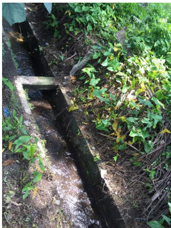
Figure 1C-30. The lined main canal of the system
