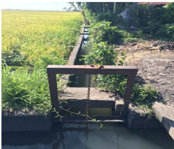
Figure 1A-108. Lateral canal without gate and lock
