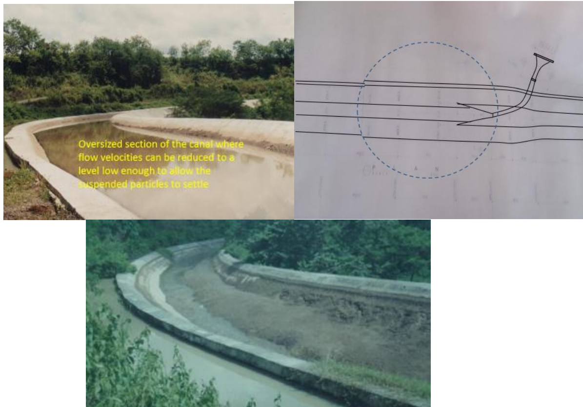
Figure 25. Settling basin at the Mlang RIS
