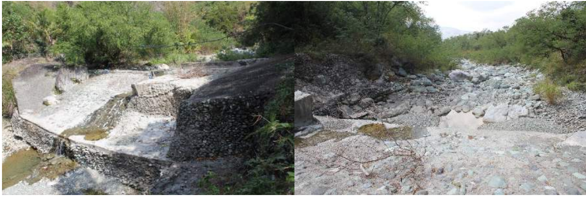
Figure 1A-28. Left: The Inasan CIS dam along the upstream of the Inasan River made of rock and concrete; Right: boulders and rocks downstream of the dam
