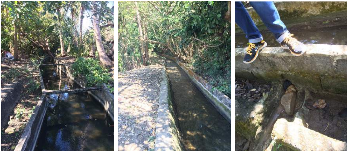
Figure 1A-65. Concrete sections of the main canal upstream (left) and midstream (middle); holes in the concrete canal serving as turnouts for distributing water to laterals; rocks are used to control the flow from the canal (right).
