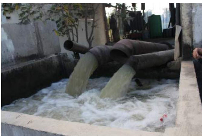
Figure 1A-4. The concrete sump where the discharge pipes of the 3 pumps empties before distribution to the main canal; the middle pump is being repaired; the water is sediment laden
