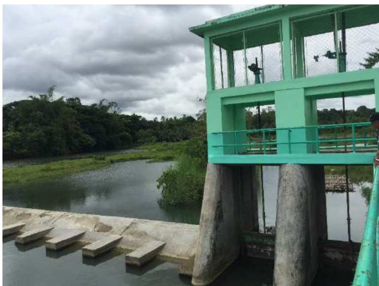
Figure 1B- 14. Two steel gates of the dam which measured 1.5 m each
