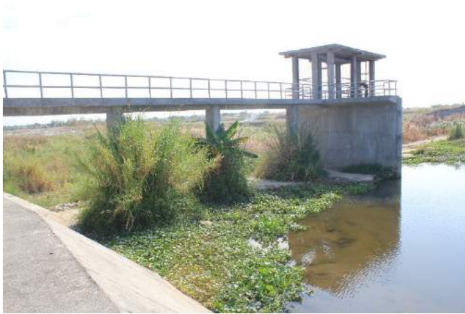
Figure 1A-13. Front view of the Anao CIS showing the heavily silted upstream portion of the dam
