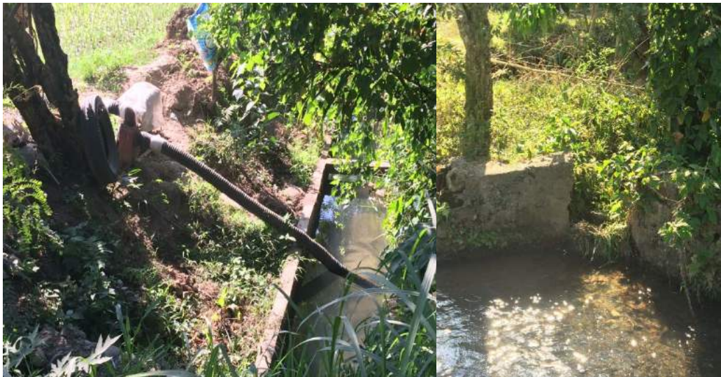
Figure 1A-75. Portions of the main canal with illegal pumps (left) and improvised lateral turnouts (right)
