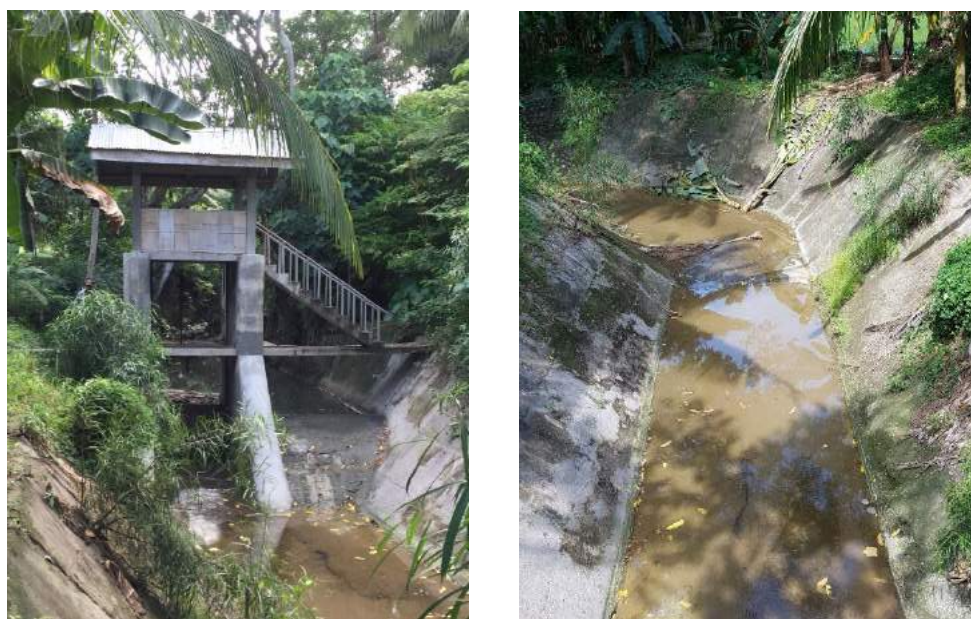
Figure 1C-8. The dam of Butilon CIS with the extended apron and side wall
