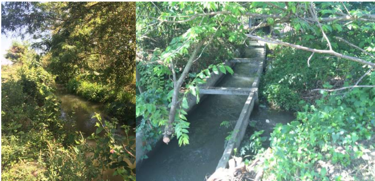
Figure 1A-73. Left: unlined portion of the main canal; Right: lined portion of the main canal with illegal turnout
