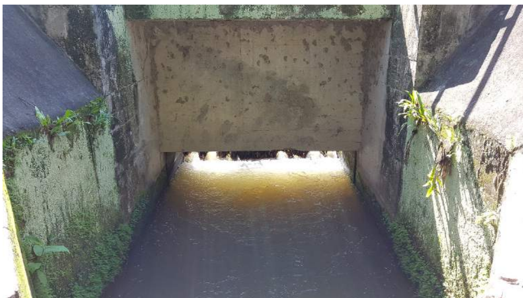
Figure 1C-26. The intake gate that is permanently open
