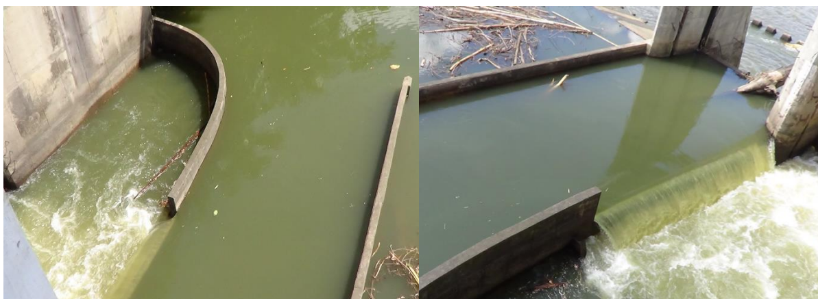
Figure 23. Construction of silt excluder at the MalRIS
