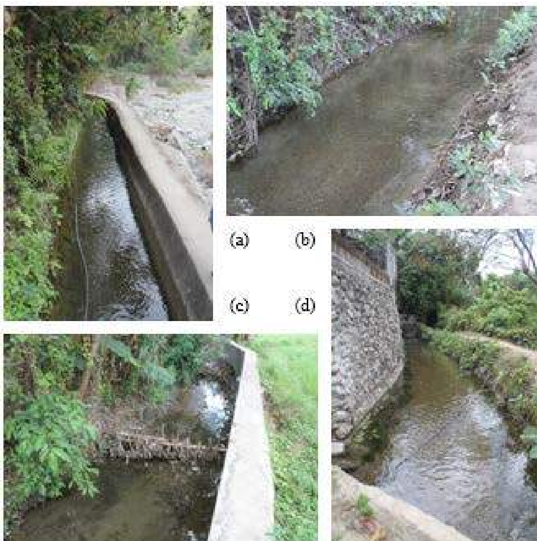
Figure 1A-53. (a-d) Pictures of the canal system with some having concrete lining, some have ripraps and most are unlined; most canals exhibit heavy siltation
