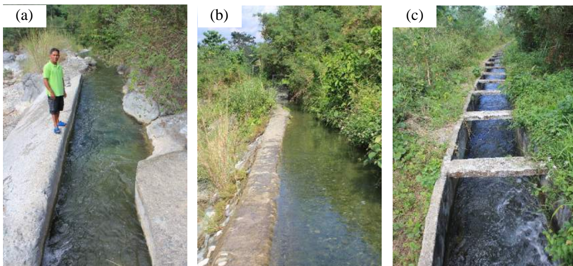
Figure 1A-39. (a) Intake channel at the side of the river just after the dam; (b) continuation of the intake channel; (c) the main canal just after the check gate Source: Author's capture
