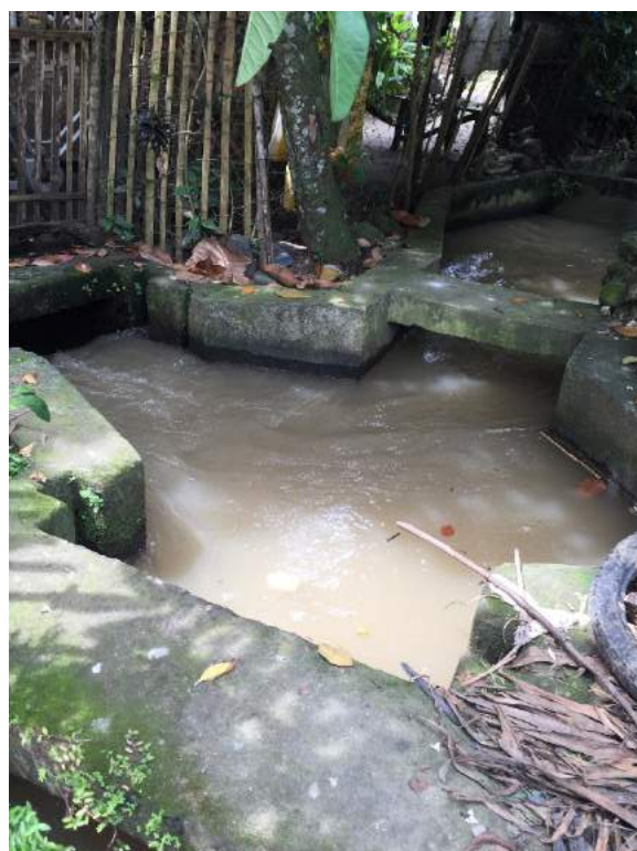
Figure 1C-20. The main canal and division box to divide flow from to different zones
