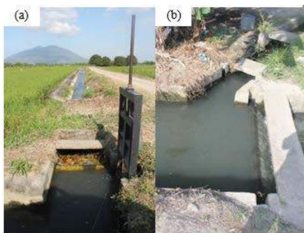
Figure 1A-19. (a) A check gate that serves as a turnout for distributing water to a secondary lateral; (b) a flow dividing structure to a lined lateral; the control has slots for wooden slabs and combined with a shallow drop
