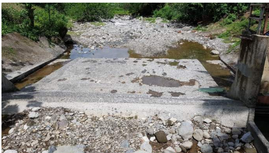
Figure 1C-33. The damaged downstream apron of the dam
