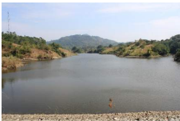
Figure 1A-45. The reservoir of the San Angel SRIP; also shown are the rocks lining the slopes of the upstream face of the dam
