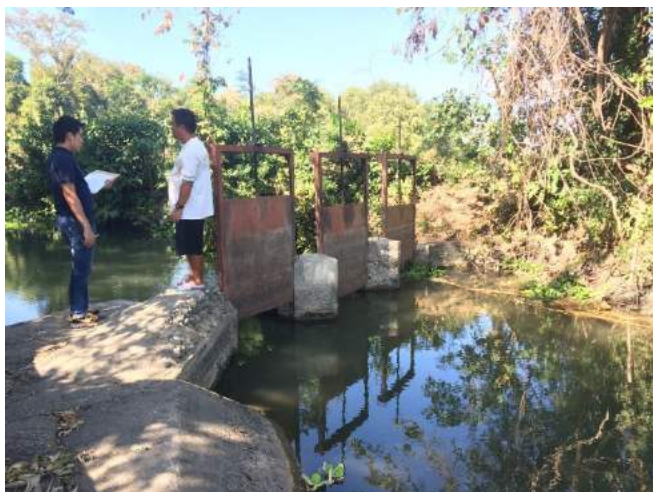
Figure 1A-59. The intake structure of the dam
