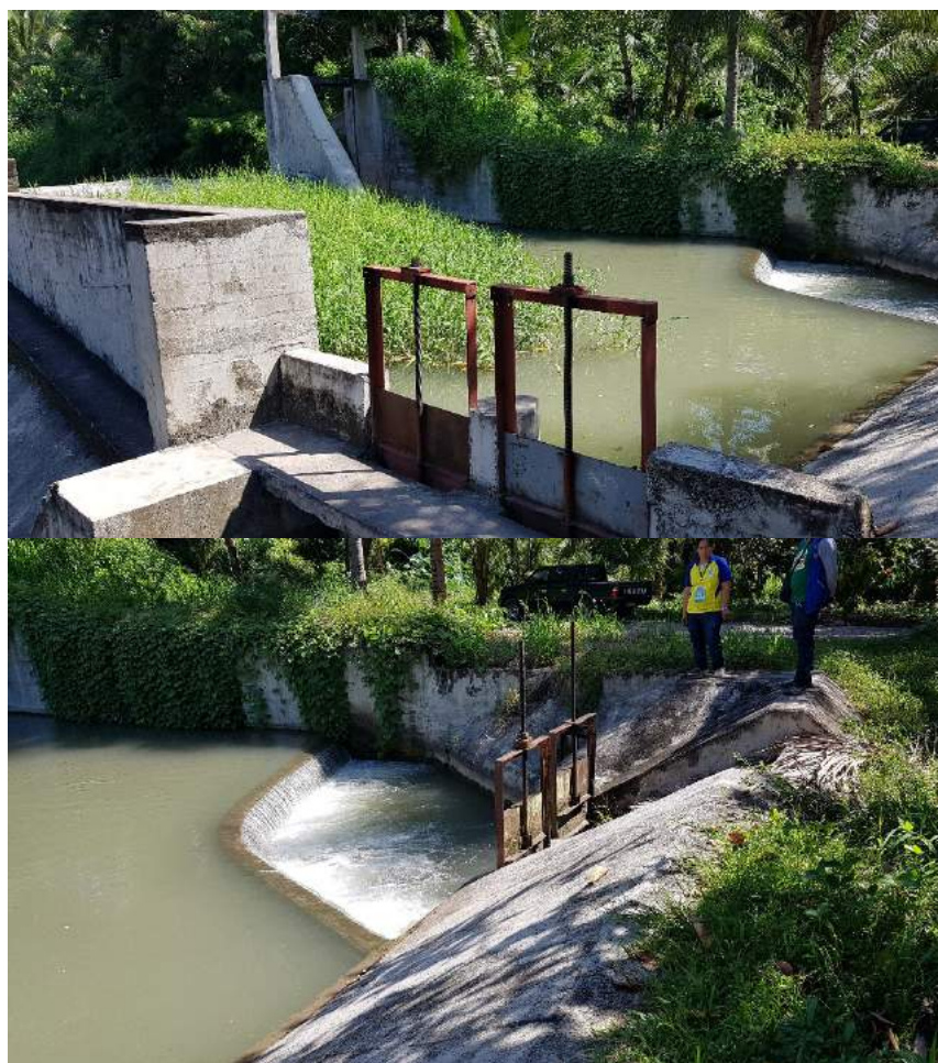
Figure 1C-23. The silt control structure and intake gate
