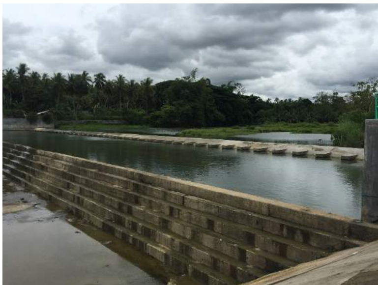
Figure 1B- 13. The diversion dam of Tagbawto CIS with a width of 100 m
