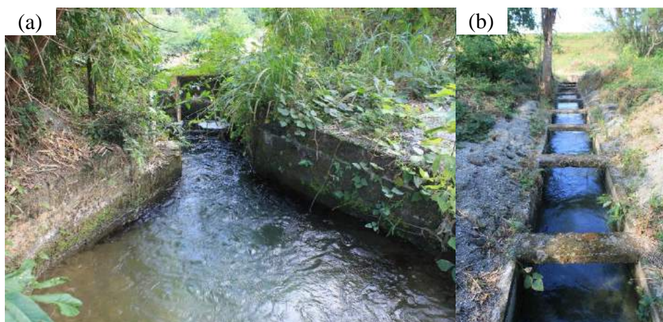
Figure 1A-42. (a) Outlet of the inverted siphon under the river; (b) the concrete-lined lateral canal after the outlet of the inverted siphon used to distribute the water to Parang-Bugnan CIS area across the river
