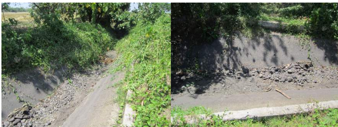
Figure 1A-96. The trapezoidal lined main canal, shown with some sediments at the bottom
