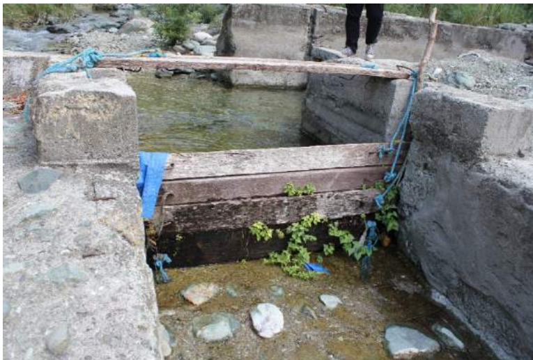
Figure 1A-29. The sluice gate is made of wooden slabs stacked together in a slot serving as water level control gate
