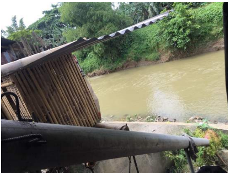
Figure 1B- 34. The 6" suction pipe used in drawing water from the Mambusao River
