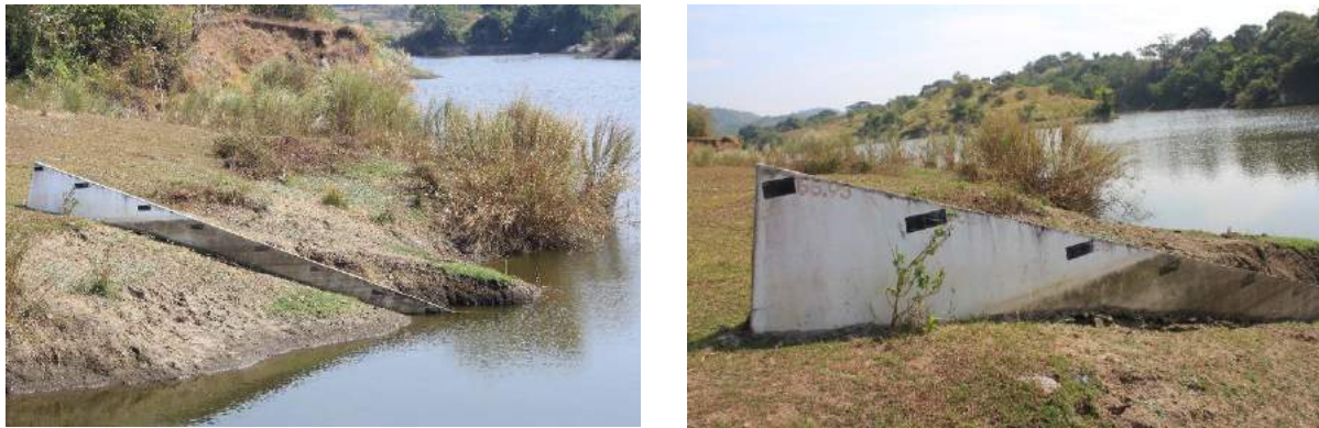
Figure 1A-46. The water level gage meter made of concrete reservoir of the San Angel SRIP; also shown are the rocks lining the slopes of the upstream face of the dam
