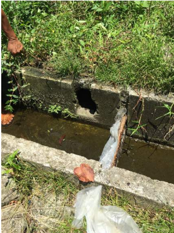
Figure 1C-31. Simple hole turnout and improvised gate
