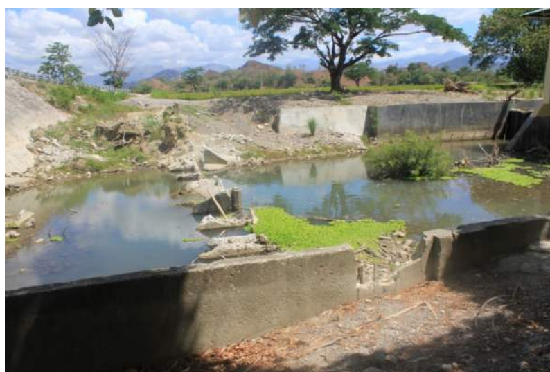
Figure 1A-115. The former Batasan CIS dam that was broken Source: Author's capture
