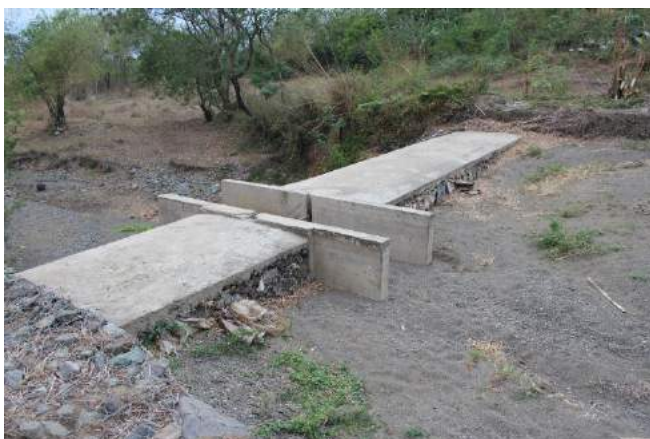
Figure 1A-23. There is no water in the creek during the time of visit and the sediments are almost up to the dam crest
