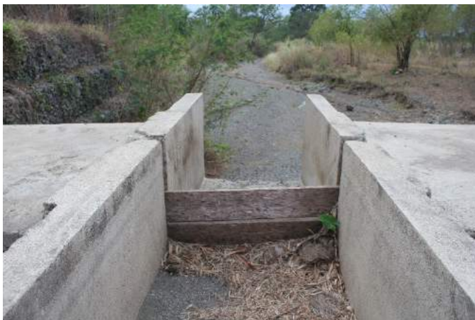
Figure 1A-25. The sluice gate is made of concrete with slots for wooden slabs serving as gates; the background is the downstream portion of the dam
