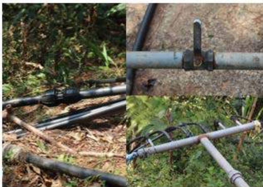
Figure 1A-85. Sample of the union patentes, gate valves and improved distribution assemblies of the Taloy Sur CIS
