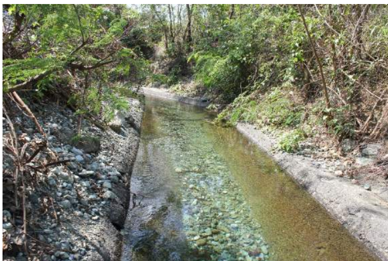
Figure 1A-33. The trapezoidal main canal; the canal bottom is filled with small rocks
