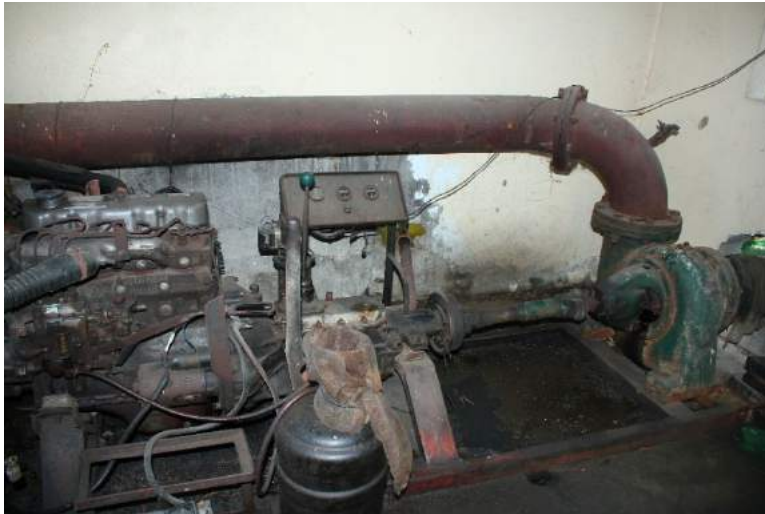
Figure 1A-8. The 8-in dia. centrifugal pump powered by a 4DR5 diesel engine of the Sapa-San Vicente PIS
