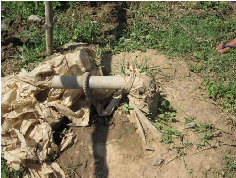
Figure 1A-92. One of the STW units; covered with plastic is the installed 4" PVC pipe, tee and reducer; visible is the 3" discharge pipe where the rubber hose of the pump is attached
