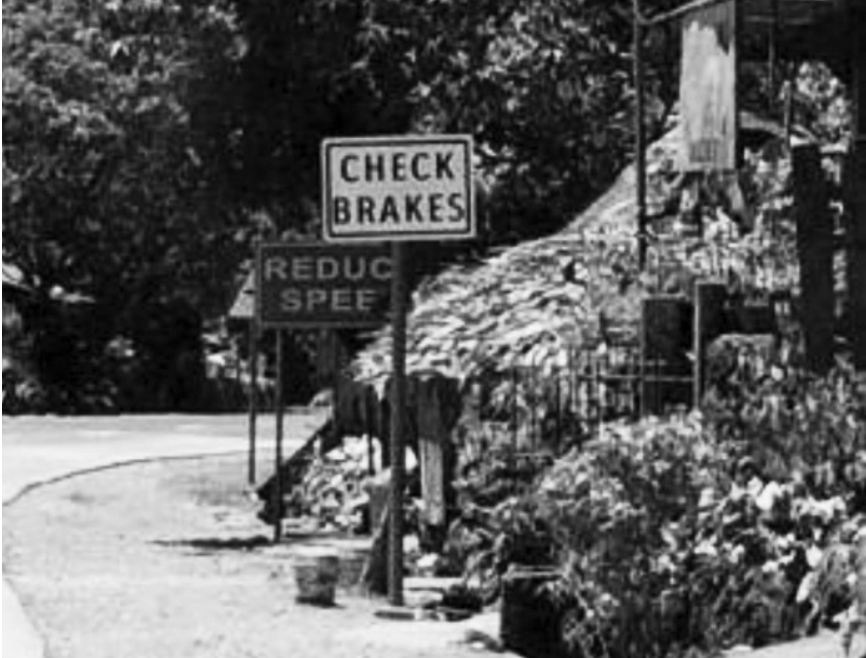
Figure 15. Imprecise arrangement of traffic signs
