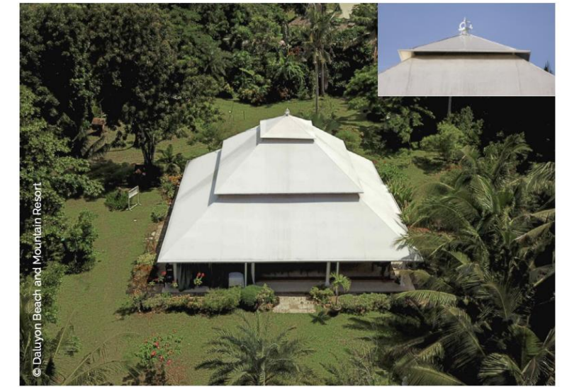
The newly installed water sprinkler at the roof of the tent.
