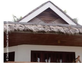
Louver ventilation installed on the roof of a guest room
